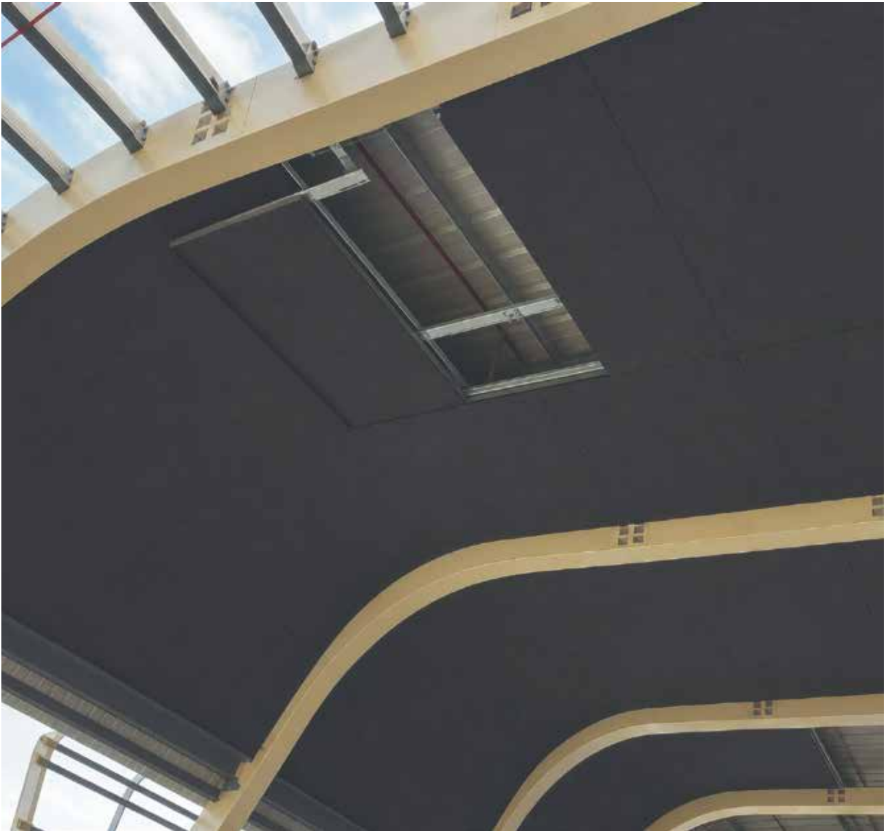
Bursa Metro Station, Türkiye
